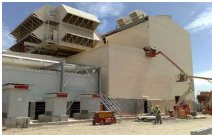
Gas1 Turbine Hall Cladding Erection
