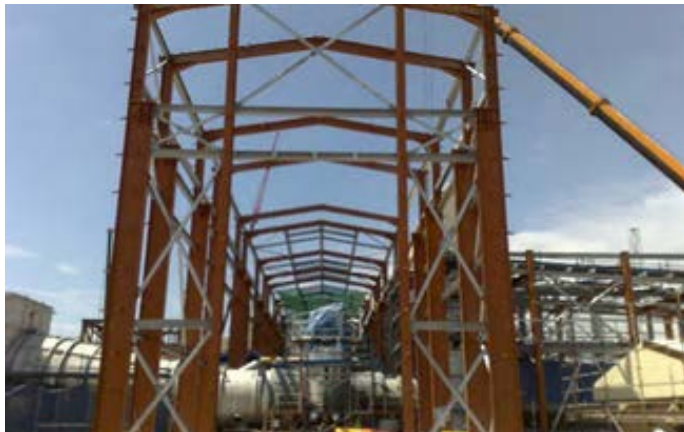
Gas1 Turbine Hall Structural Steel Erection
