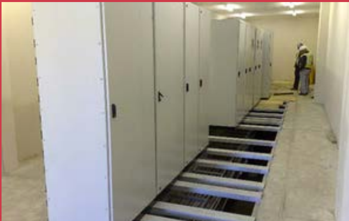
MCC Cabinet Installation
