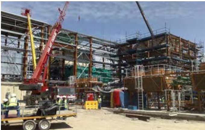
Gas1 Turbine Hall Structural Steel Erection
