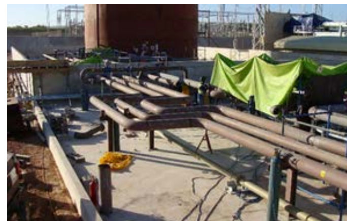
Fuel Piping Under Construction
