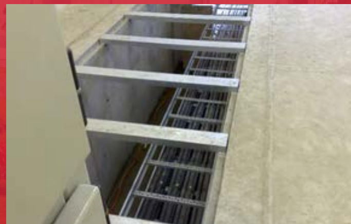
Cable Installation in The MCC Room
