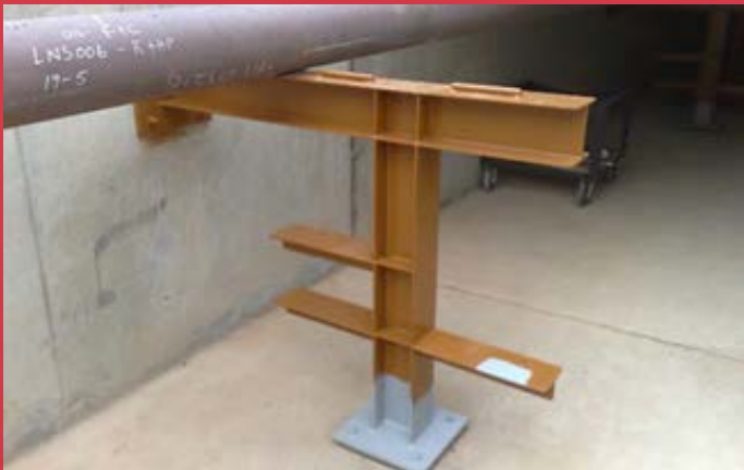
Siemens Piping Installed on Supports
