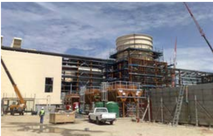
Gas1 Turbine Hall Cladding Erection
