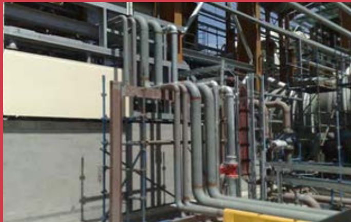
Siemens Piping Installation
