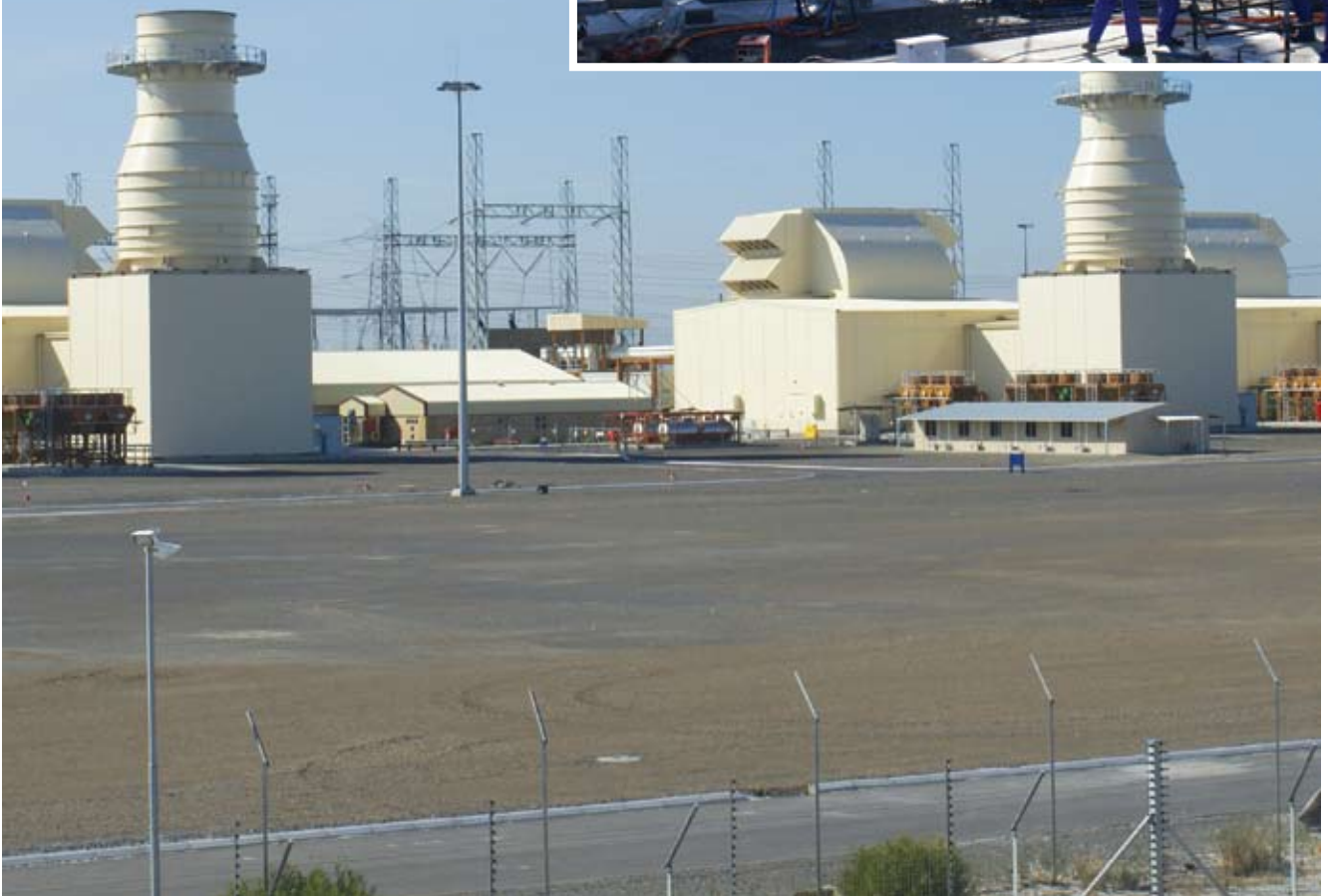
Completed OCGT (Open Cycle Gas Turbine) Project in Atlantis Cape Town
